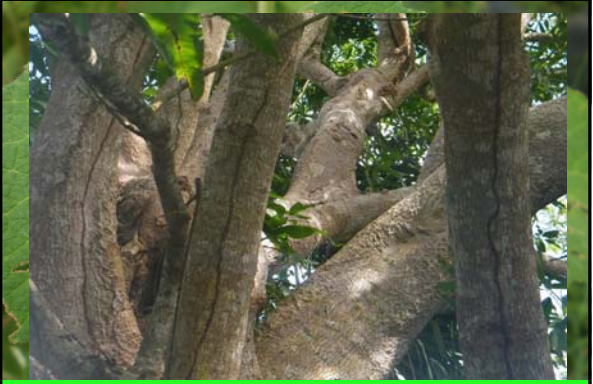
Termite ( Coptotermes gestroi ) pathway "mud galleries" on a tree
